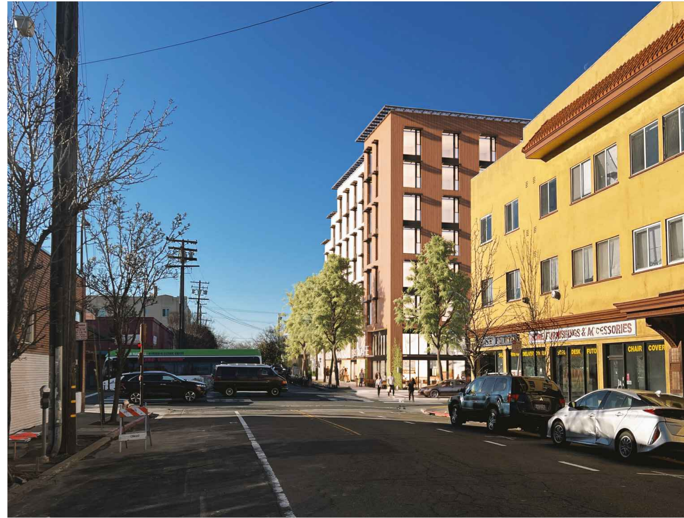
2 CALIFORNIA LOOKING SOUTH - AFTER
